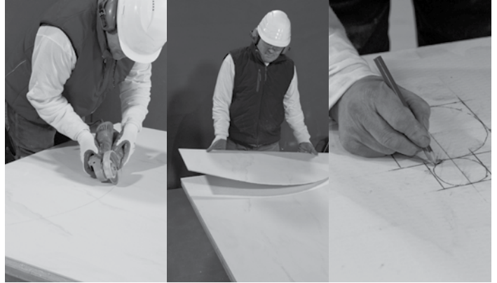
Cutting and holes
