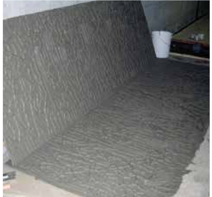
Example of proper full mortar coverage
