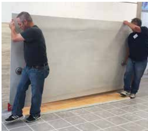
Example of suction cup handles being used. Panel weight is approximately 140 lbs. and no more than 2 experienced people are suggested to move.
