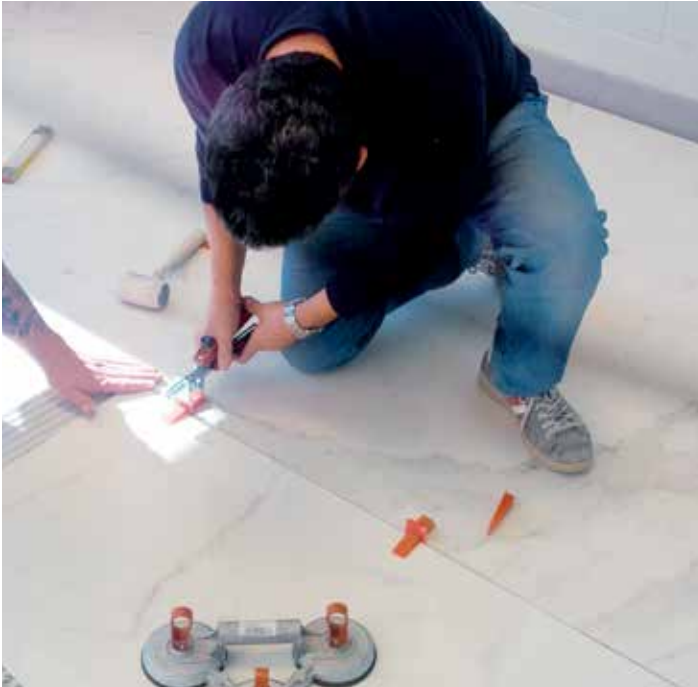
Self-leveling system being used for floor installation
