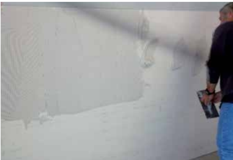
Example of full skim coat being applied
